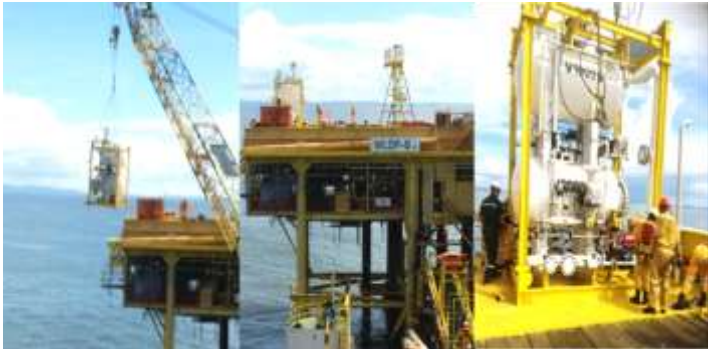
SEP-iSYS™ LPPU Lifting and Installation on WLDP-B.
