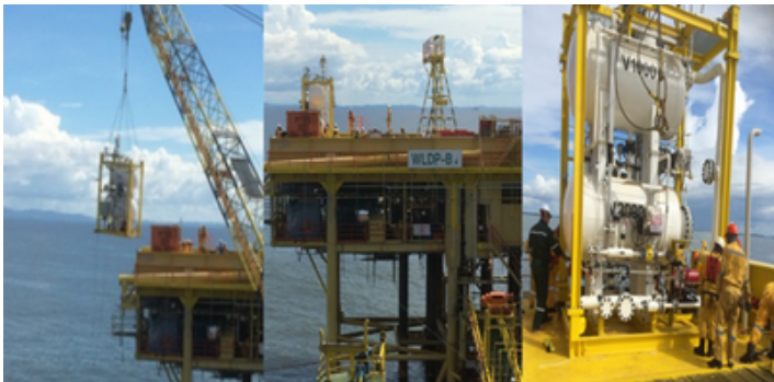
SEP-iSYS™ LPPU Lifting and Installation on WLDAP-B.
